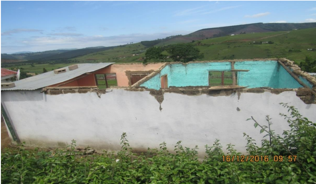
Figure 48: House destroyed by heavy wind
