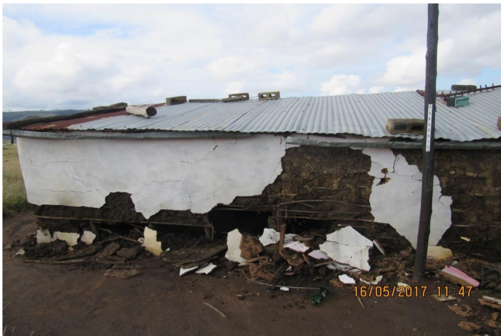
Figure 50: House destroyed by heavy rain
