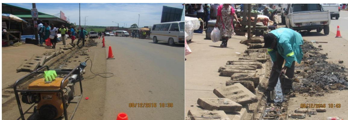
Clearing of storm water drains
